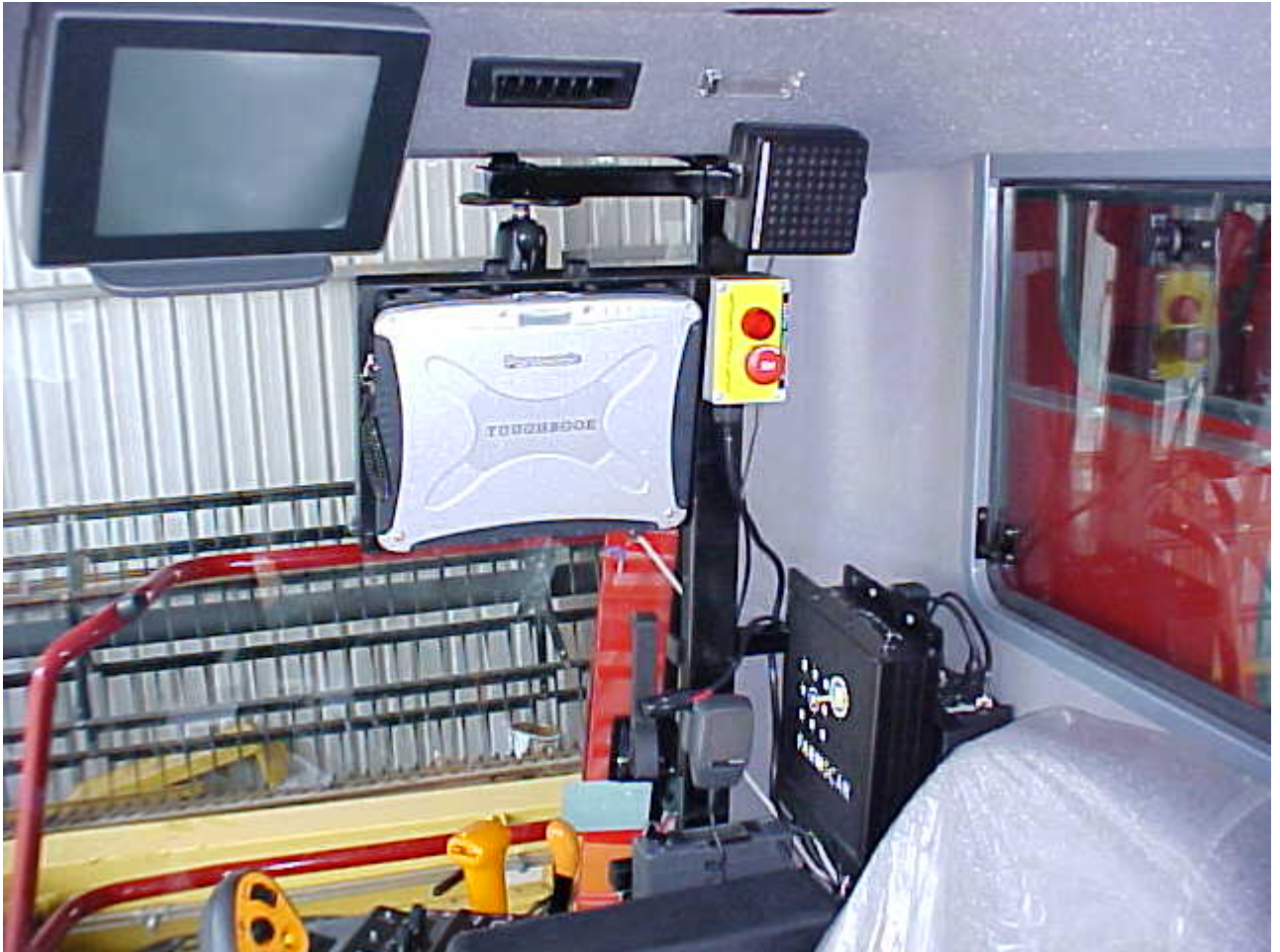
In Cab installation of the console
