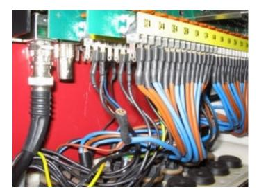
An instruction sheet on the inside of the Hardi pilot junction box lid lists the function of each wire. Disconnect relevant female connectors from the circuit board inside the Hardi junction box and connect them straight into the corresponding male terminals on the loom coming from the farmscan junction box.
