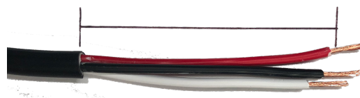
Cable should be trimmed to a minimum of 70mm for easier install in junction box
